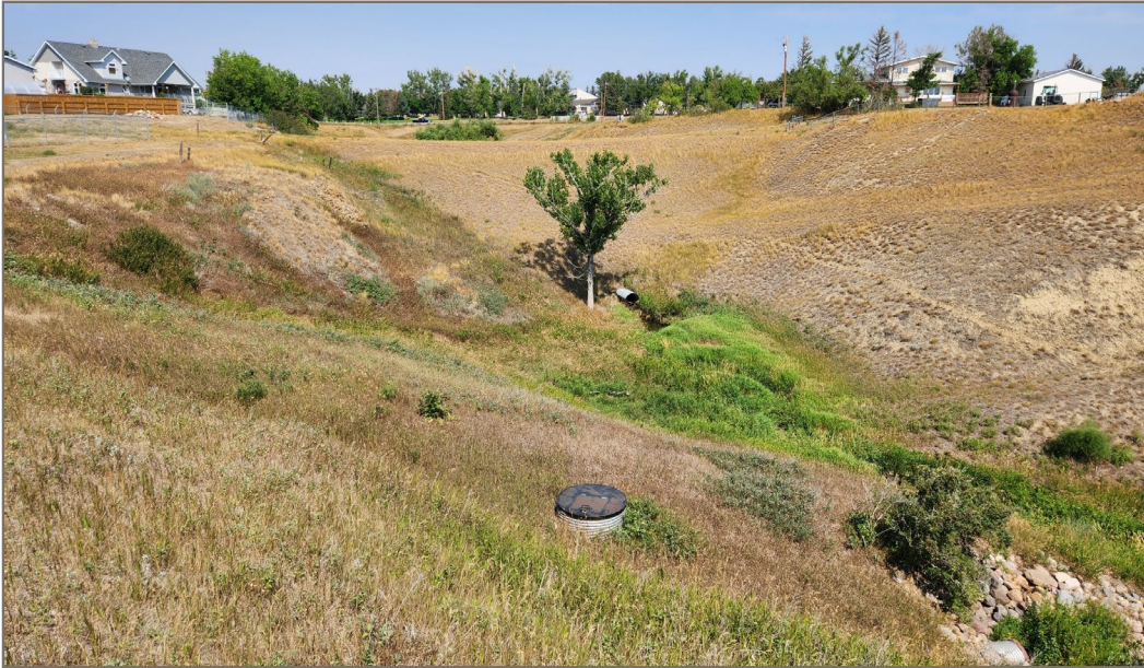
Photo 5: Culvert Upstream of the Tributary Coulee.
