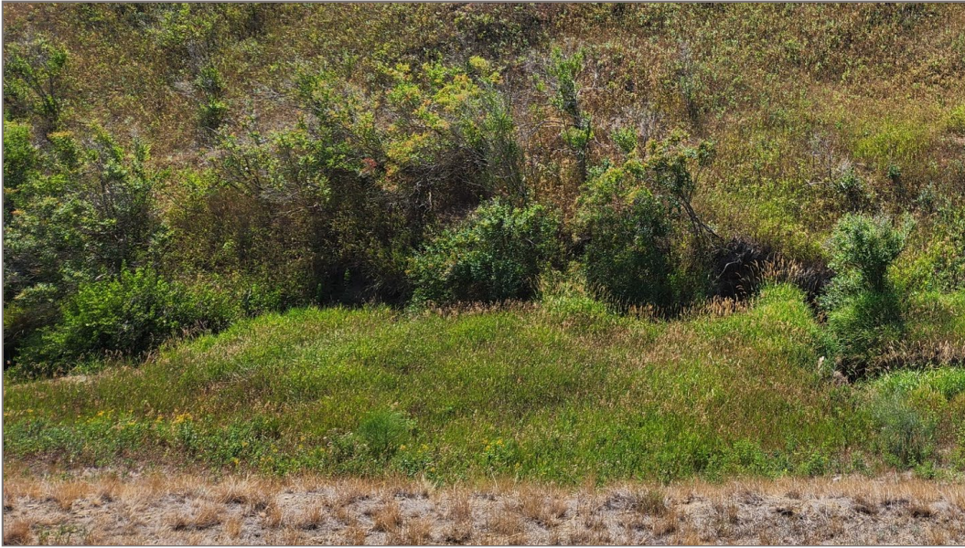
Photo 7: Channel Visible at the Toe of the Site Slope – Facing South Across the Tributary Coulee.
